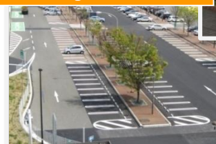
Parking lot sidewalk
